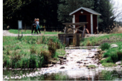
Outlet from treatment facility (WWTP and wetland) in Nynäshamn, Sweden
